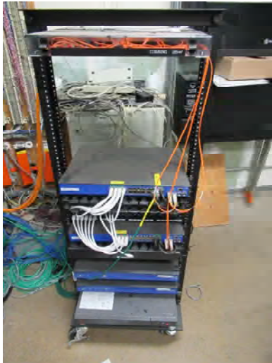
EXISTING NETWORK RACK AT 300W IDF, ROLLING RACK
